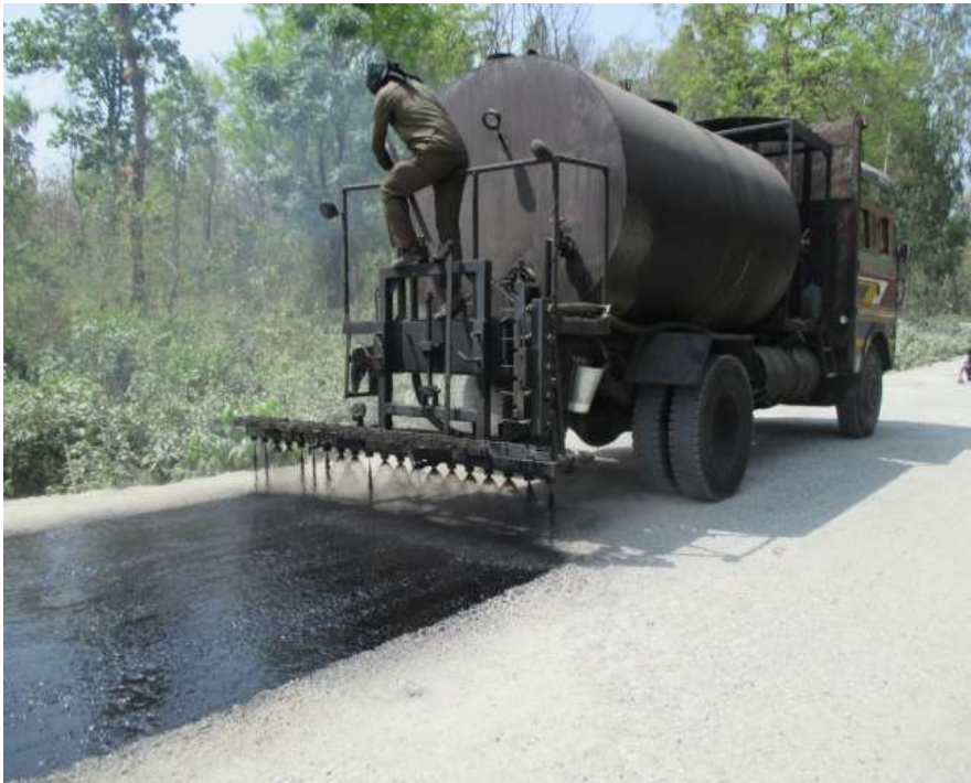
Prime coat works at K-K Road
