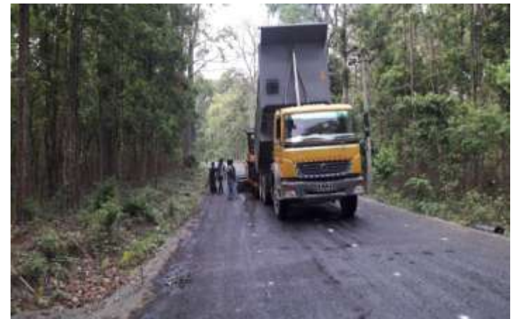
Asphalt Concrete works at K-K Road
