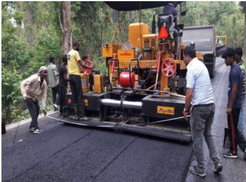
Asphalt Concreting works at K-K Road
