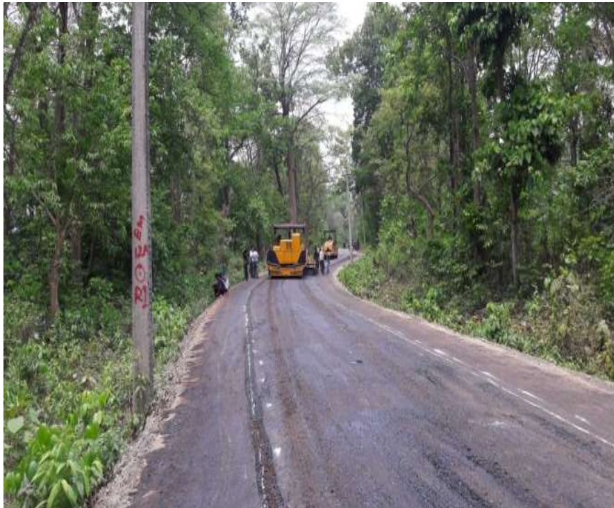
Application of Tack coat at K-K Road
