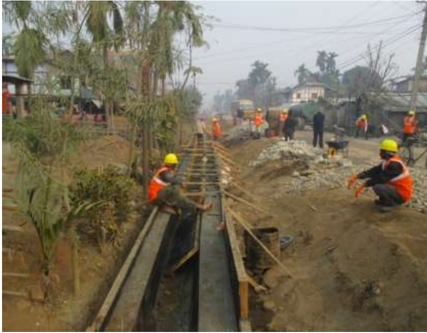
Plum concrete drain works at P-S Road
