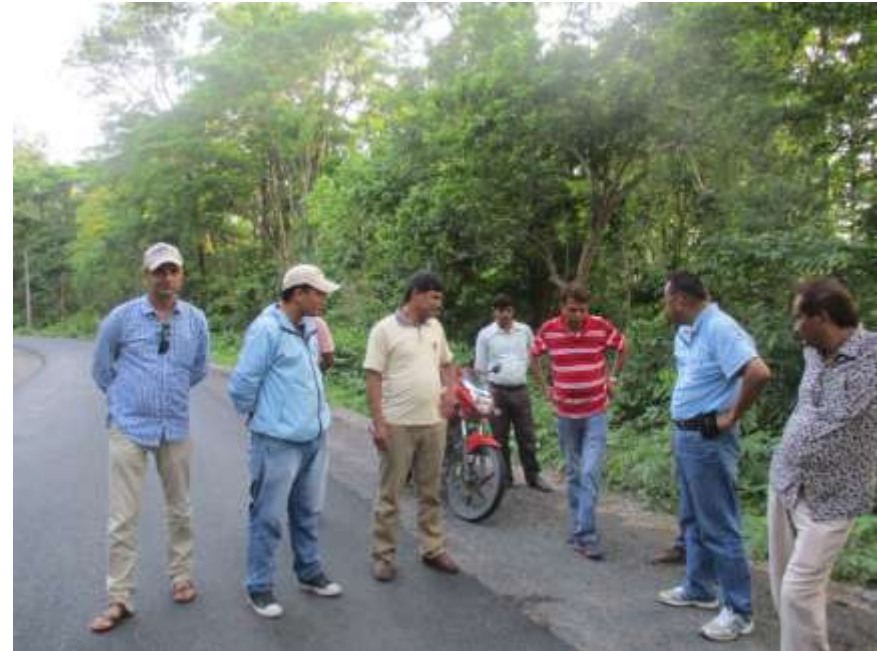
Jt. Monitoring of K-K Road by DC/ CMS/DTL/Imp. Team/Contractor after AC pavement laying
