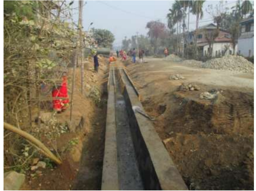
Plum concrete drain works at P-S Road
