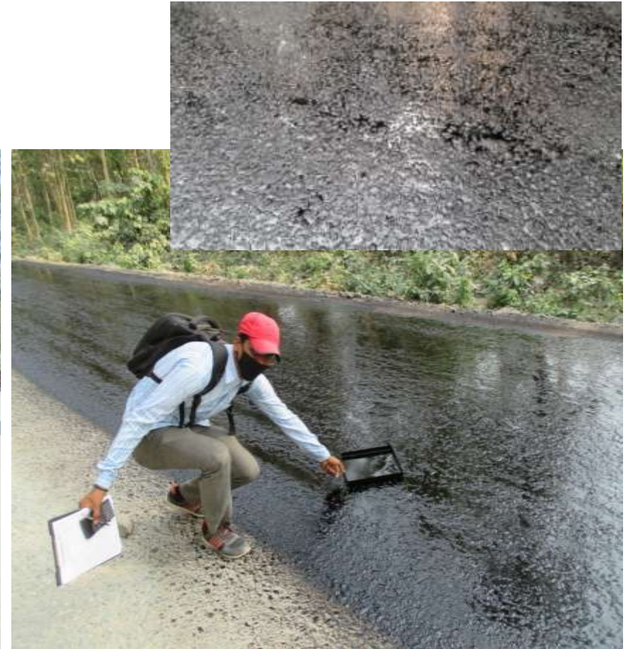
Prime coat works at K-K Road
