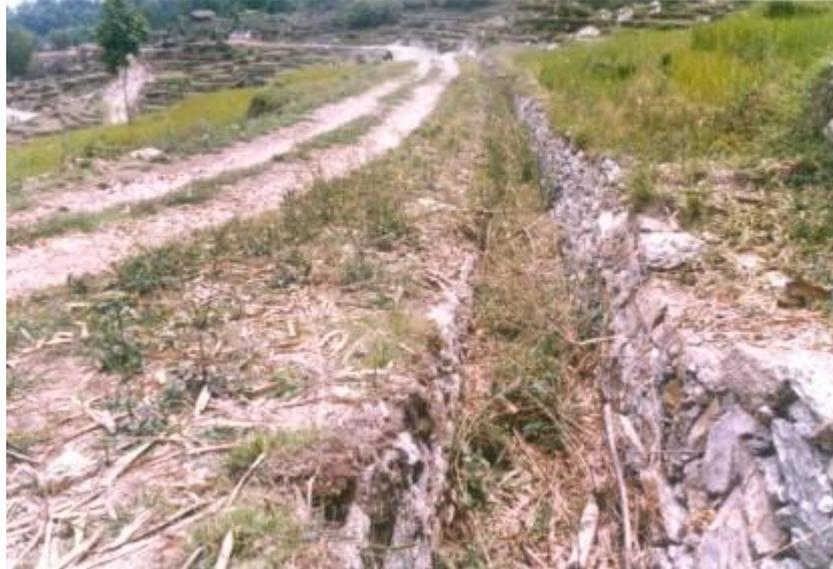
*An overfilled drain that needs to be immediately cleaned*
