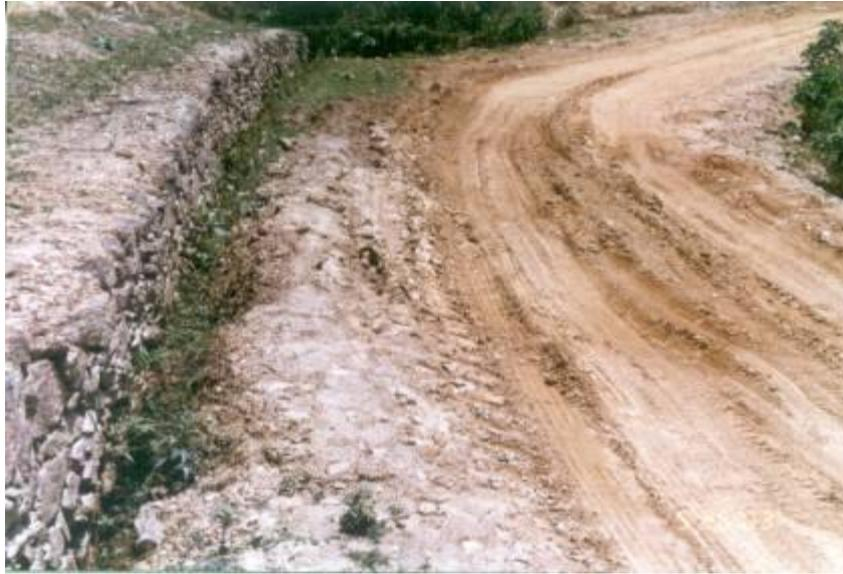
*Damaged shoulders that call for recurrent repair and maintenance*
