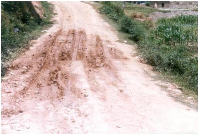
*The furrows made by motor tyres should immediately be filled up.*
