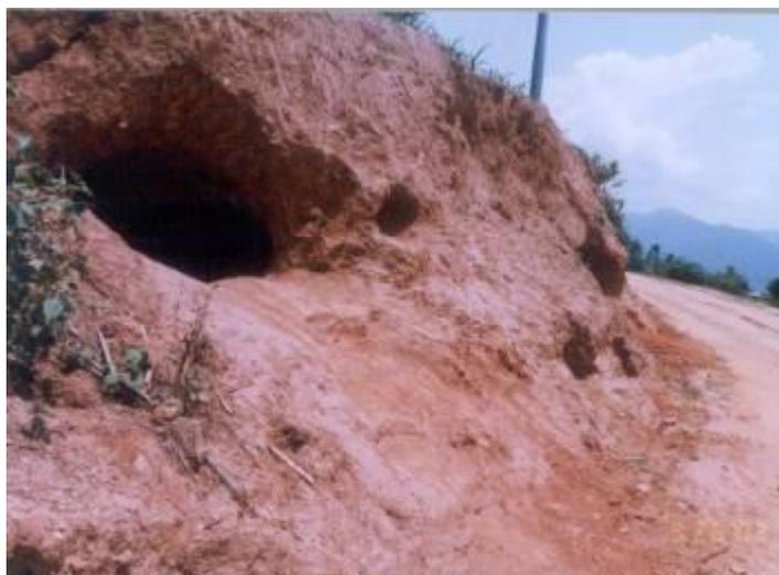
*Damage caused by excavating red clay from road edges.*
