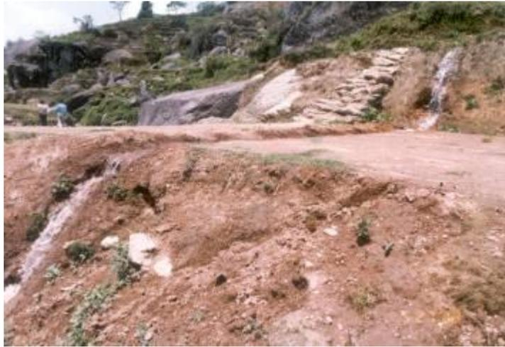
*Draining water by cutting the diagonal drain*
