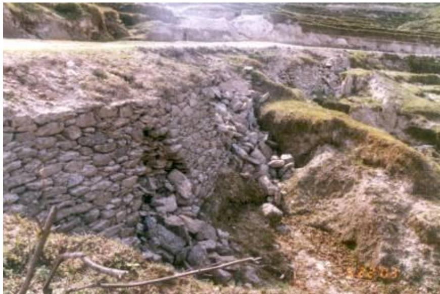
*Wall of dry stones requiring immediate repair and maintenance*
